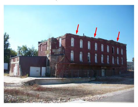
Figure 5 – Exterior view showing stepped parapet along the side wall.
