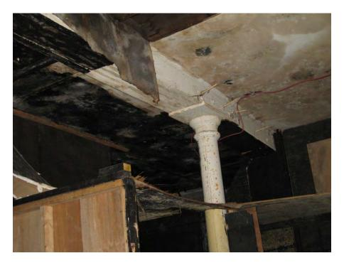
Figure 10 - Example of iron column and wood ceiling beam at the  $2^{\text{nd}}$  floor.
